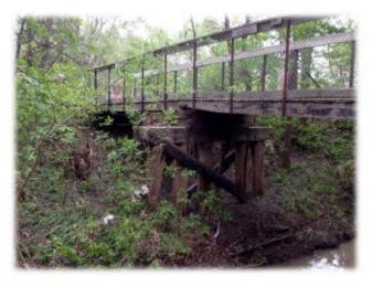
caused the bridge deck to move laterally and drop downward. Recommendations were included in the inspection report that ranged from repair of the damaged area to full replacement of the bridge.
